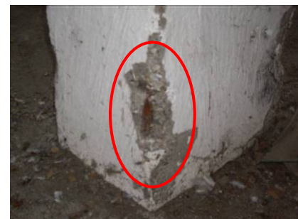
acier corrodé apparent
